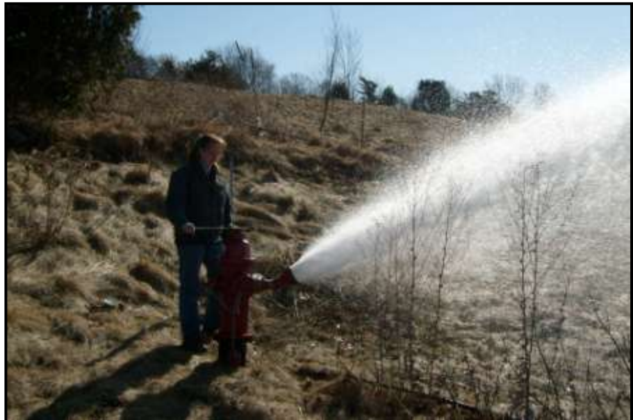
Retail employee Deb Sweeny conducts a fire flow test
