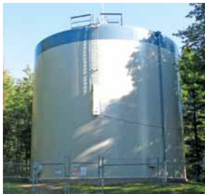
Essex North Tank (after recoating summer 2012)
