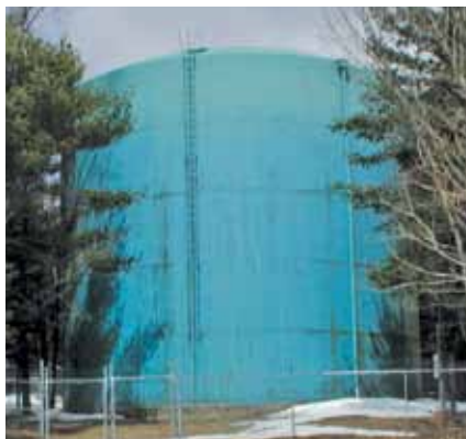
Essex North Tank (prior to recoating in 2012)
