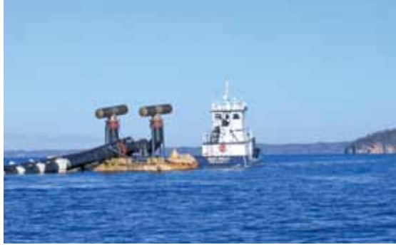
Tug boat towing south intake into position to sink in 80' of water depth (2007)
