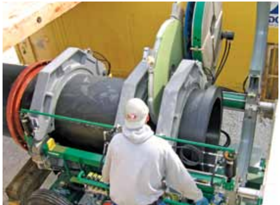
Fusion welding of high density polyethylene (HDPE) intake pipe (2007)
