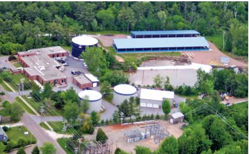
Aerial view of the CWD Treatment Facility
