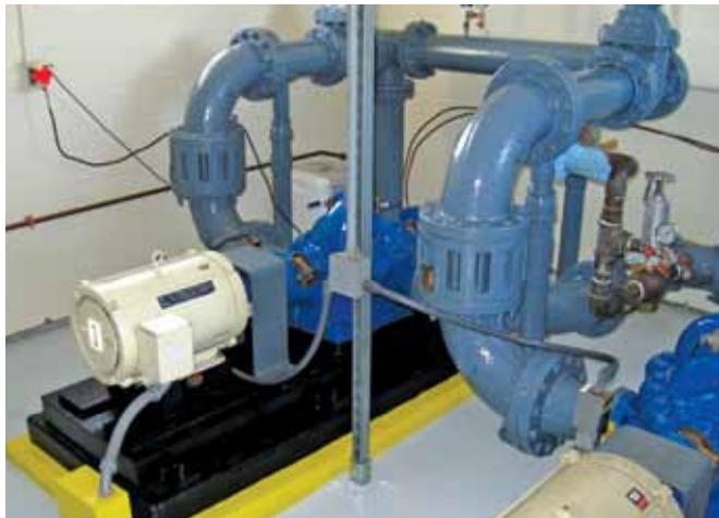
Rehab of Williston East Pump Station (2012)
