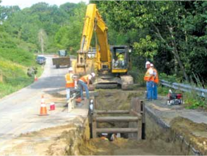
High Service Cross Tie Project trenching (2012)
